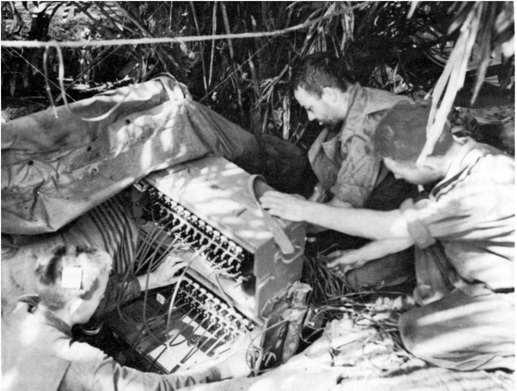
SETTING UP A FIELD SWITCHBOARD
