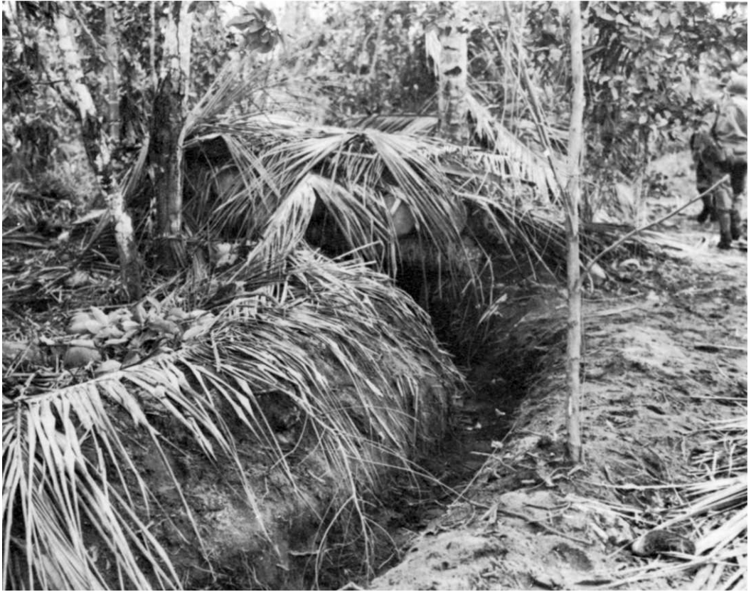
COCONUT LOG BUNKER WITH FIRE TRENCH ENTRANCE in the Buna Village area.
