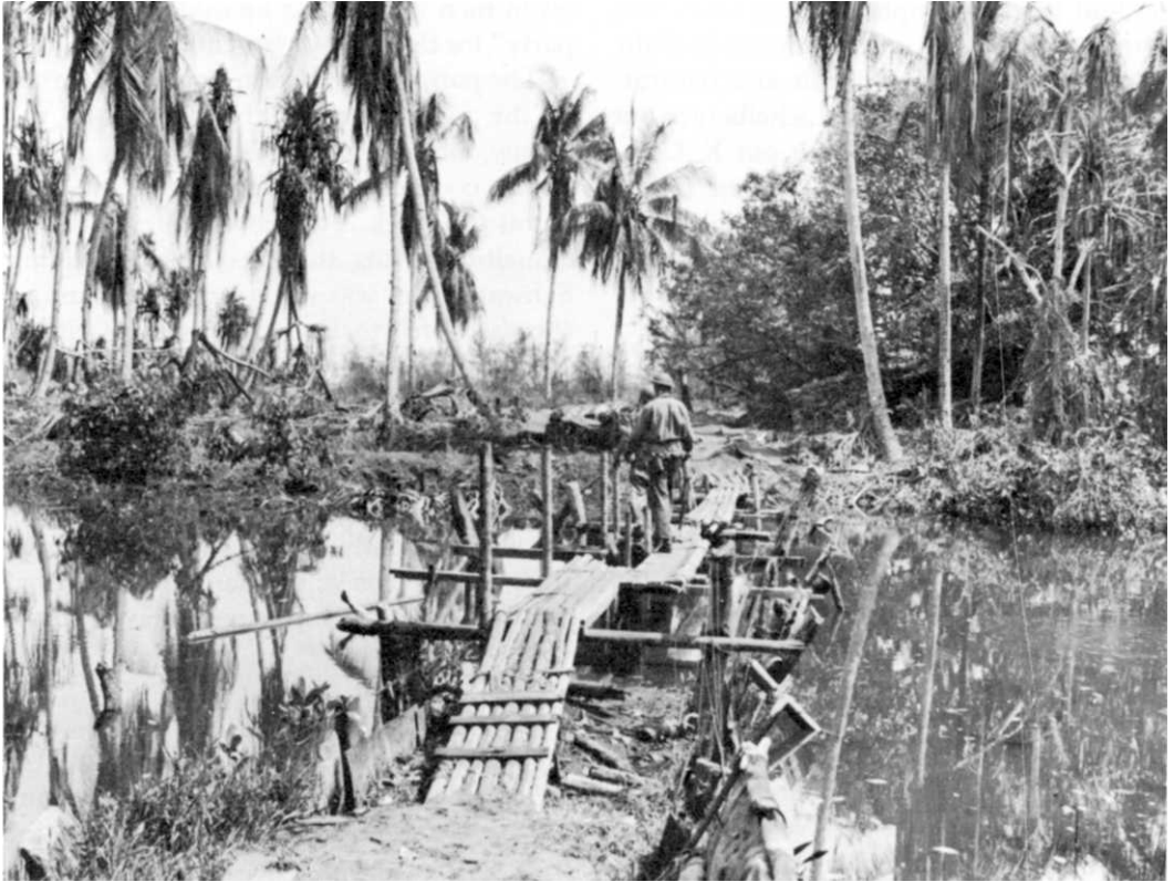
FOOTBRIDGE OVER ENTRANCE CREEK to Musita Island .
