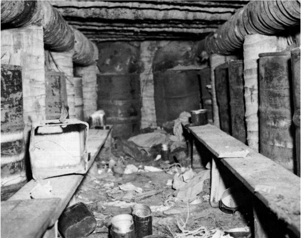
INTERIOR OF COCONUT LOG BUNKER reinforced with sand-filled oil drums near, Duropa Plantation.
