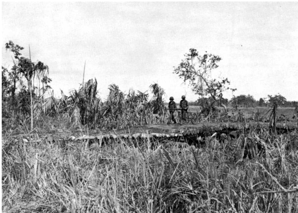
BRIDGE OVER SIMEMI CREEK. New Strip in the background. (Photograph taken after bridge was repaired by the 114th Engineers.)
