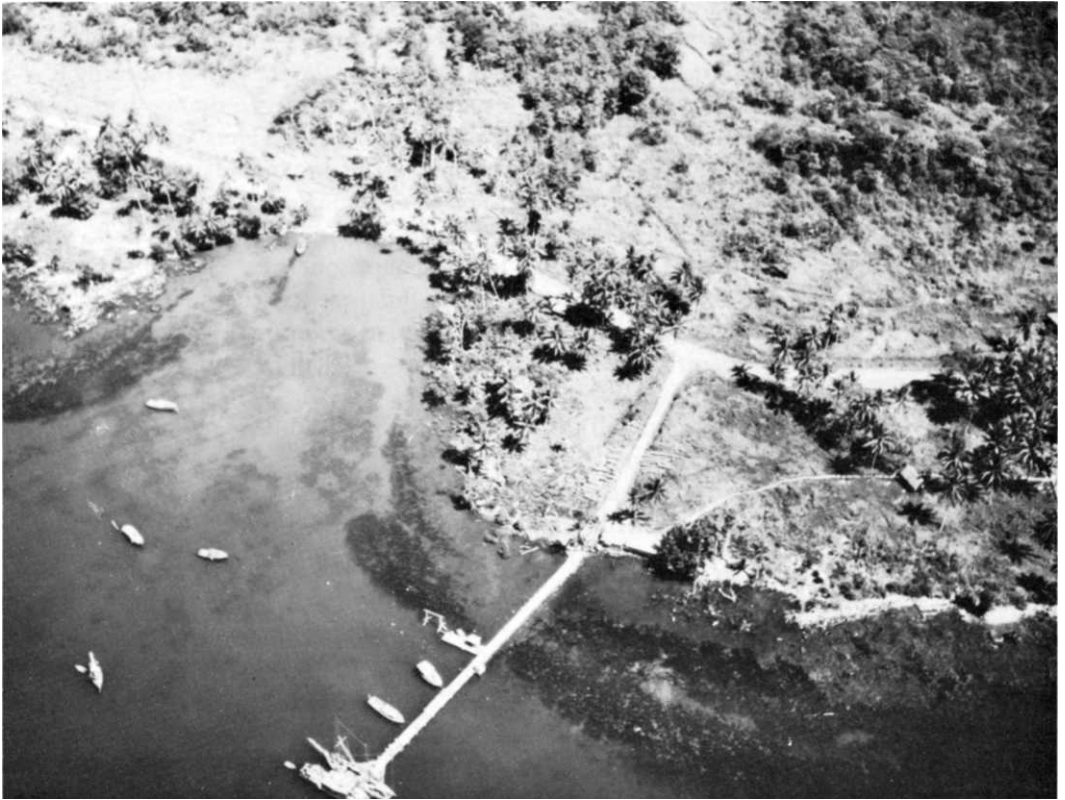
WHARF AT GILI GILI built to replace old jetty.
